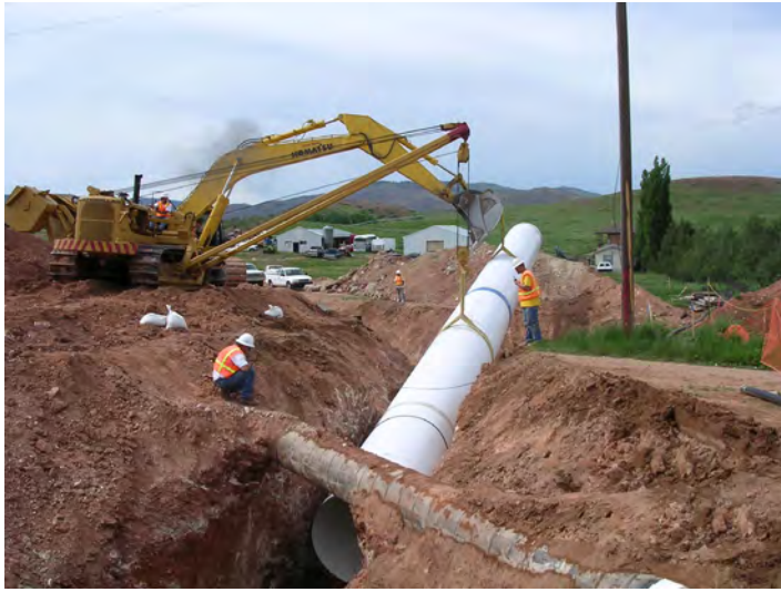
Construction of Pleasant Valley Pipeline
