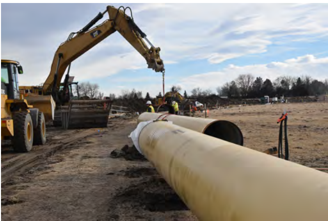
SWSP II construction in Boulder County
